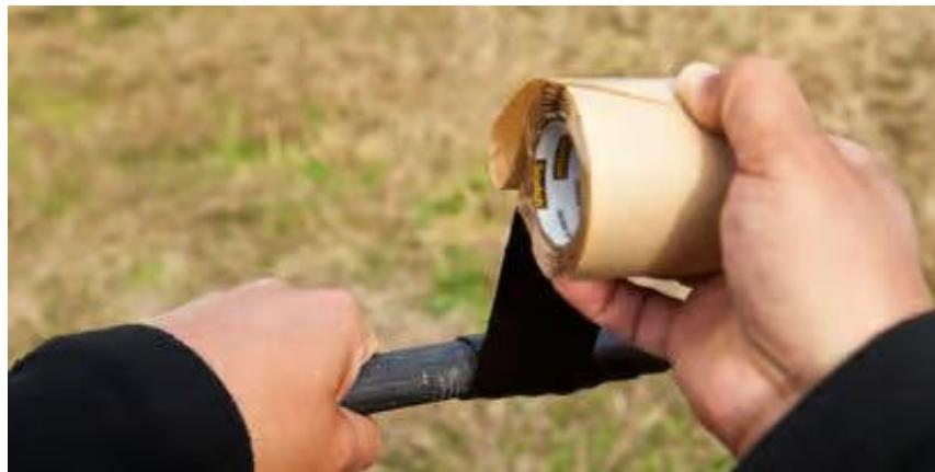
Quick, safe, and cost-effective method to restore cable protection.
